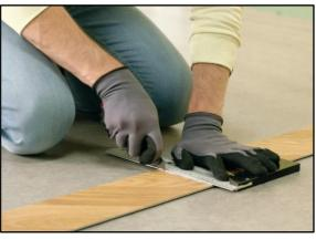
Lay the floor panel with the decor side up. Use a carpenter's square, measurer or another floor panel to cut along in a straight line. Cut with the knife two or three times over the piece to be shortened. Then turn the floor panel and break off the piece easily. Is the piece to be cut off too small? Then use a pair of pliers. If desired, you can also cut off the long piece of the panel with a hand, electric or jigsaw power tool. Replace the blades or saws if they are blunt.
