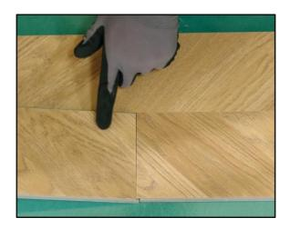
5. Place the cut floor board on the end side with the groove in the tongue at an angle of ±30 degrees and then lower it.
