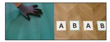
8. From the third row onwards, place the planks row by row. Make sure that you place enough spacers in the expansion joints so that the floor does not shift. Use a varying mix of decors and planks from different packs. In each row there are either all A planks, or all B planks. Each row alternates between A and B.
